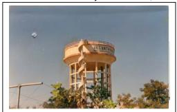
separate septic tank for the colony, an overhead tank of 1,25,000 gallon capacity and an underground water tank fitted with a pump having capacity of 2,50,000 gallon for supply of drinking water to all houses. The Society also constructed two way 60 feet wide main road, whereas all internal roads were 33 feet wide which were later on handed over to the Municipality for
